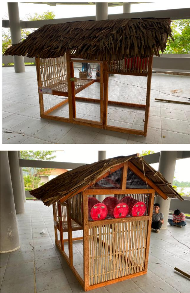
Fig. 3 – Modular Poultry Chicken Coop with a Knock-Down System
